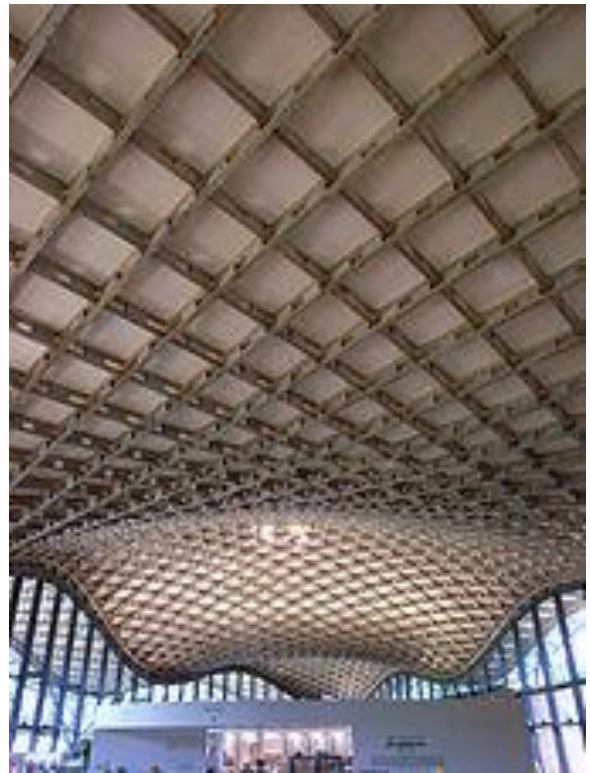
Savill Building, the wooden gridshell roof.
