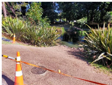
10: Soil leveled and rolled
