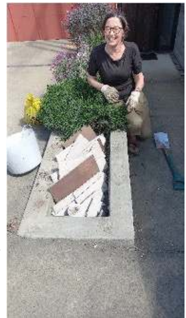
Fig 3. Placing the tiles
